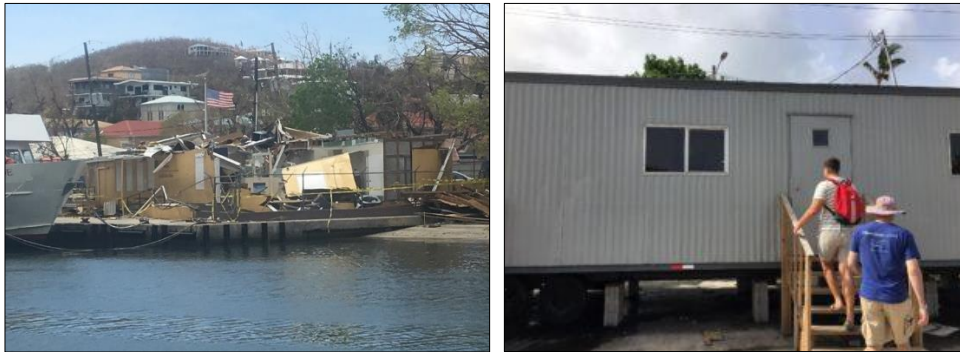
The U.S. Customs Facility in Cruz Bay was completely destroyed. A temporary trailer now houses the CBP operation at the Victor Sewer Facility with a permanent replacement expected in April 2019.
