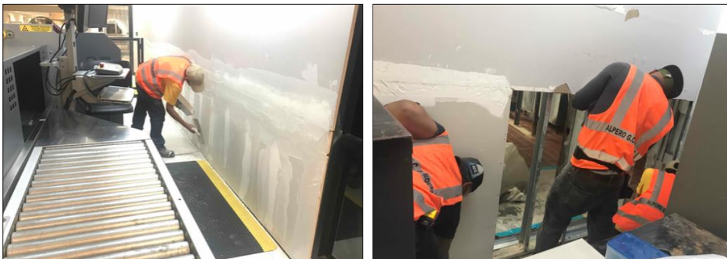
Now that the CEKA Terminal roof is almost completed, travelers will notice a significant improvement to the appearance of the interior of the terminal in the upcoming weeks.
