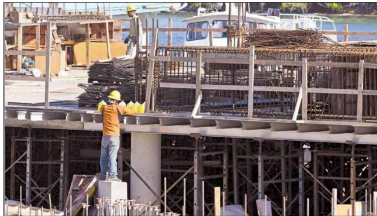
The Red Hook two-level parking garage should be completed by December 2018.
