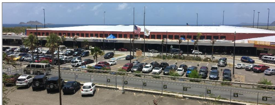
The entire roof of the CEKA Terminal is being replaced, with expected completion by November 2018.
