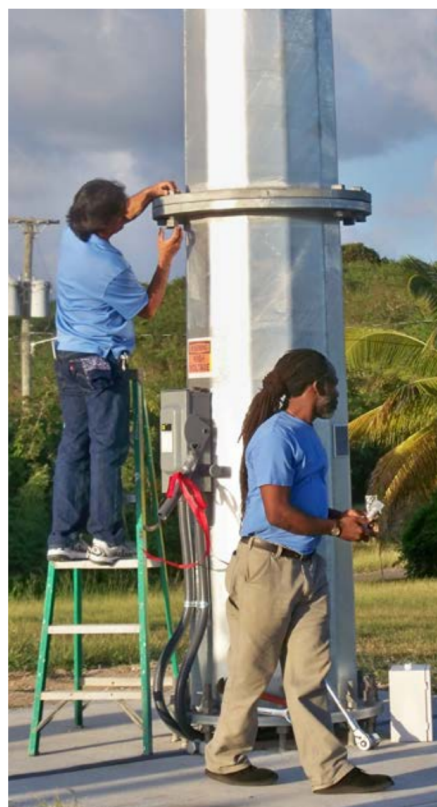
Workers install a 10-kilowatt wind turbine at the St. Croix Reformed Church and Kindhill School in St. Croix. Photo from Don Buchanan, VIEO, NREL 20418
