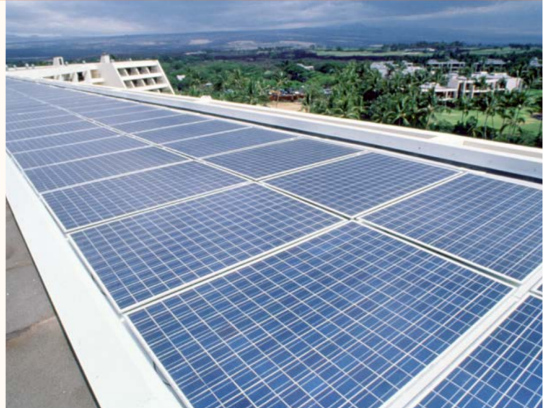
The rooftop solar PV on Hawai‘i’s Mauna Lani Bay Hotel generates 75 kW of electricity. Photo from SunPower, NREL 06430
