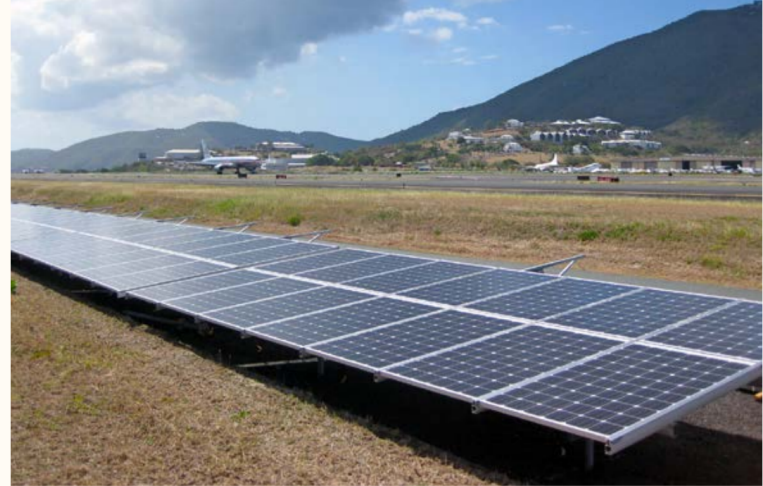
A 448-kW PV system installed at the Cyril E. King Airport on St. Thomas in April 2011. Photo by Adam Warren, NREL 18953
