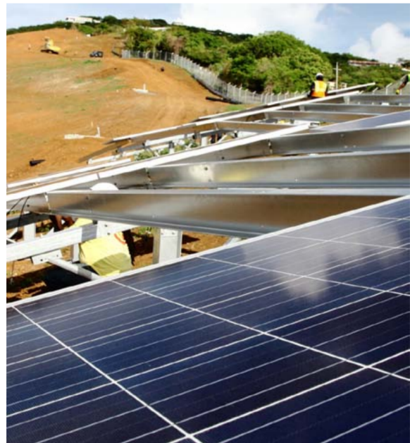
Estate Donoe Solar Project on St. Thomas
