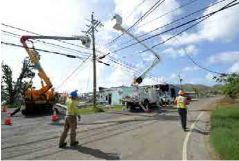
Crews working on power restoration Source: FEMA
