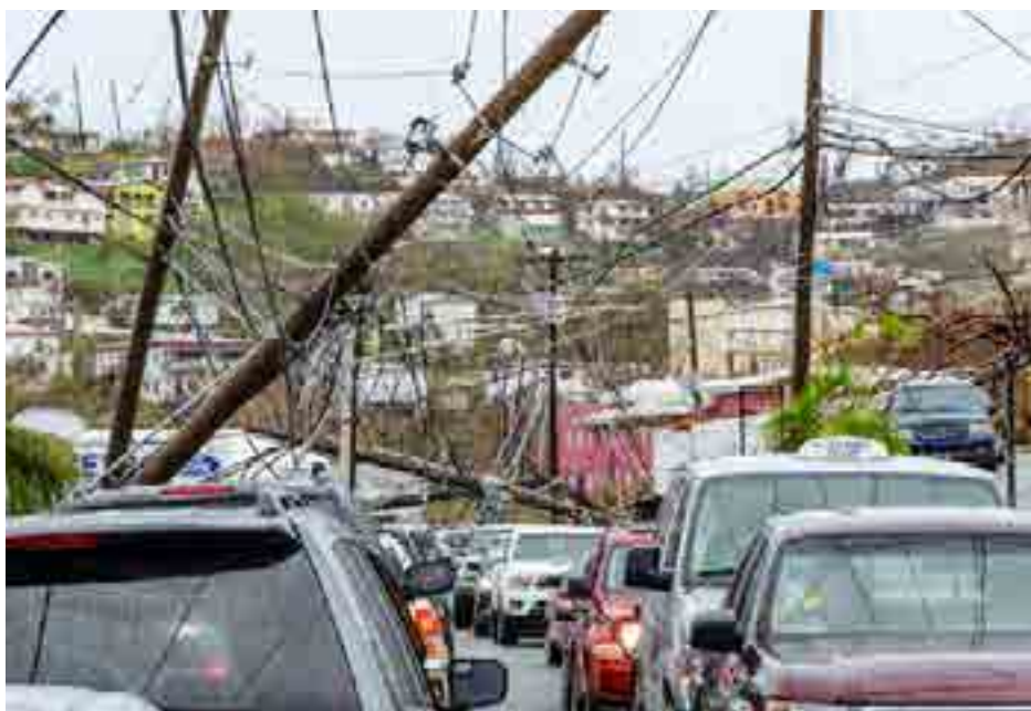
Hurricane damage to power lines in St. Thomas, Source: Kenneth Wilsey/FEMA
