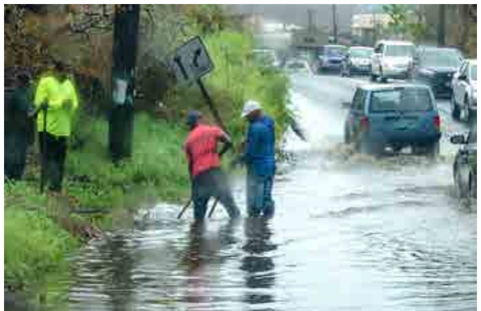
Workers clear debris from roadside drains during a rain storm to alleviate flooding on St. Thomas. Source: FEMA/K.C. Wilsey
