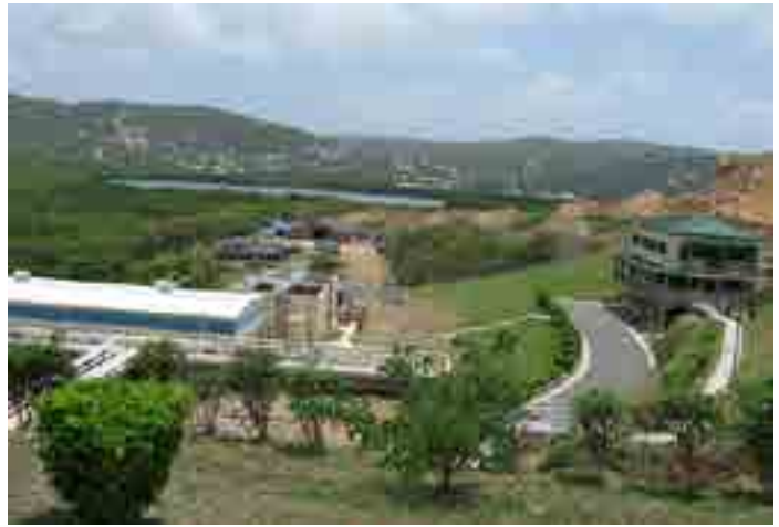
Mangrove Lagoon Wastewater Treatment Plant; Source: VIWMA
