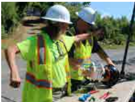
Repairing Source: viNGN
